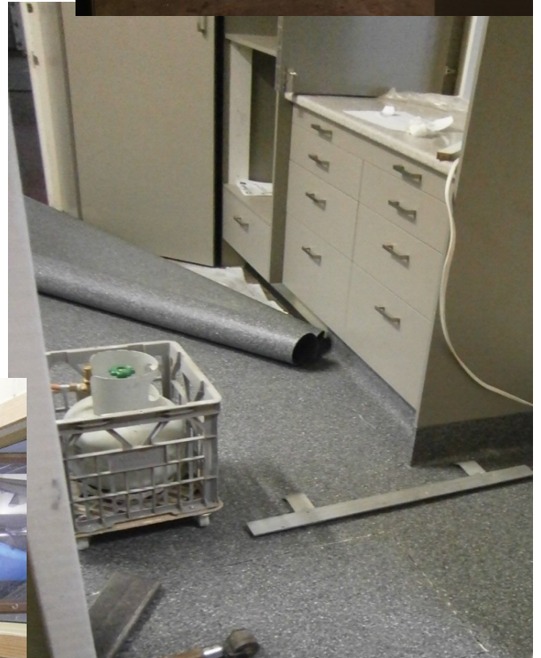
Vinyl Flooring almost in place !!!
